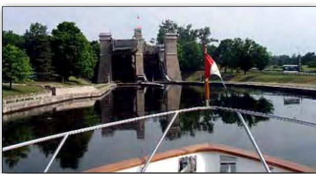
Peterborough 65 foot vertical lift lock. The water in each chamber weighs 1,500 tons (330,000 gallons). An extra foot of water is added to the upper chamber (130 tons) which forces it down and the lower chamber up.
