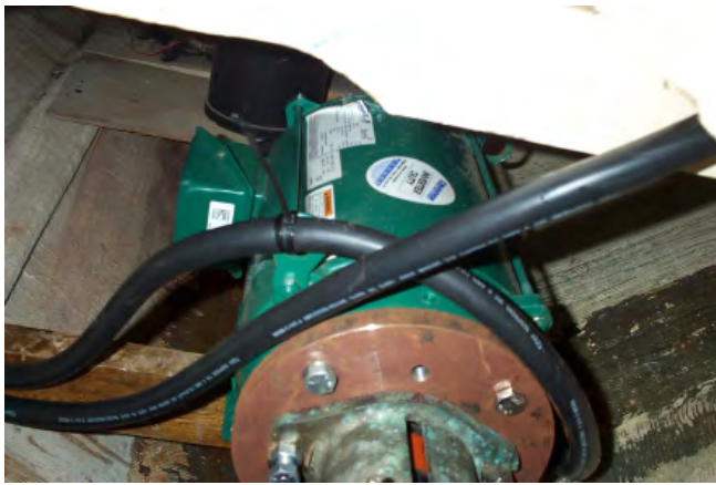
View of motor and adaptor plate
